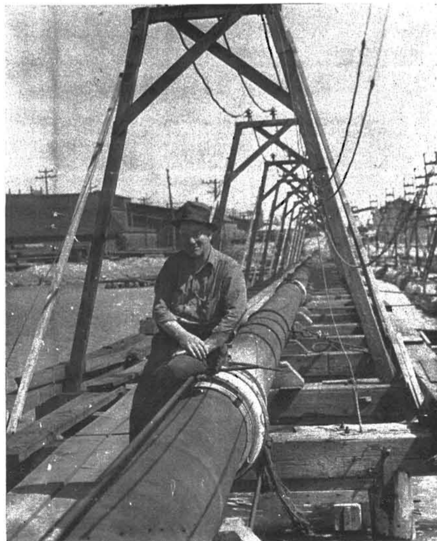
Dredge discharge flows through these pipes to Storage Pool at Shore Plant. Note overhead power line; also the genial Master, Oliver Baril, who has had charge of dredge and discharge lines throughout the thirty years of operation.
